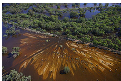
Breach in North Loddon River levy © DSE Victoria
