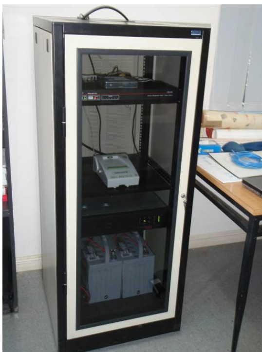
Figure 11: Power options; solar primary installation and pack-up battery installation
